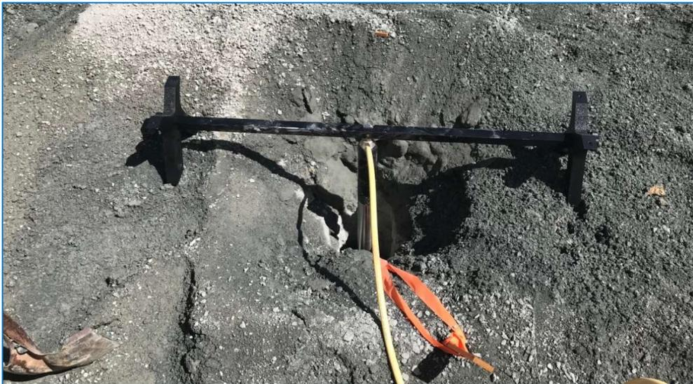
*Figure 37 Vertical alignment with end-pieces in place*
